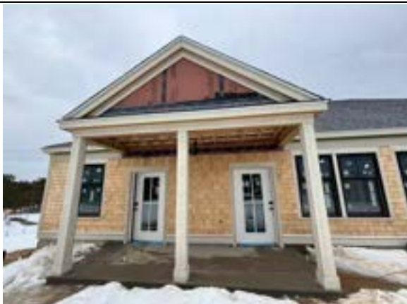
Photo 8.5. The exterior of the east wing is nearing completion.
