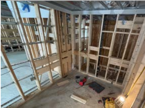
Photo 8.11. Rough MEP work has started in the common restroom.
