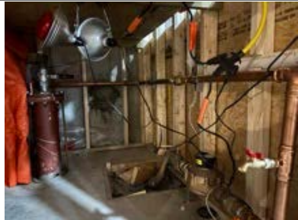
Photo 8.12. Rough plumbing has progressed in the basement.
