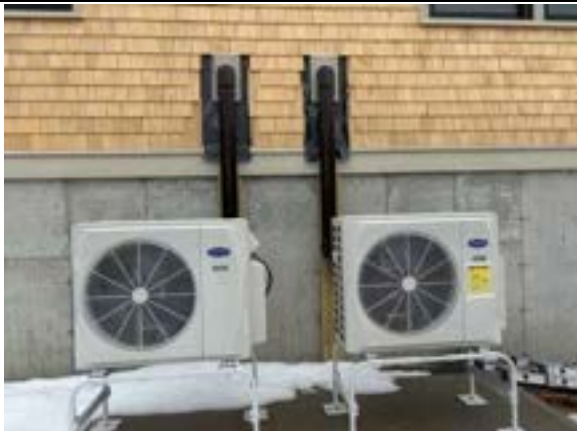
Photo 8.3. Outdoor condensing units, refrigerant lines and wall penetration progress.
