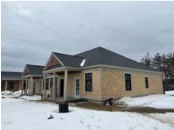
Photo 8.1. The exterior of the north wing is nearing completion.
