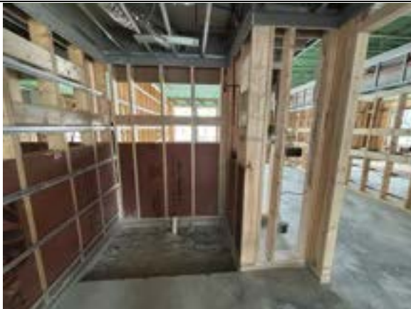
Photo 8.17. North wing concrete slab has been cut to coordinate shower drainage.
